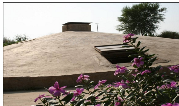
AG Community Tank, Gram Tank
